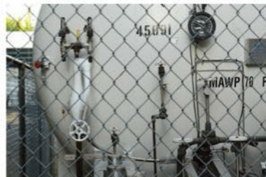
Difficult inspection sites
